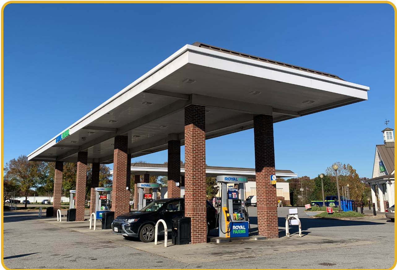
Above: Canopy lighting located at 1201 South Church St. The canopy lighting illuminates directly below the canopy, preventing excess light from escaping into the night sky.
