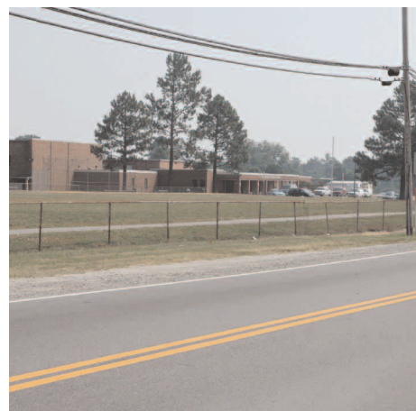
Chain link defines school property.
