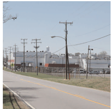
Large industrial building with shallow setbacks.
