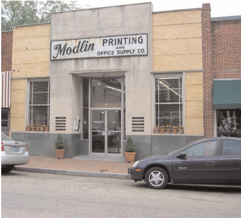
A variety of building materials and textures help to articulate this facade. Integral brick bands contribute to the buildings horizontal expression.
