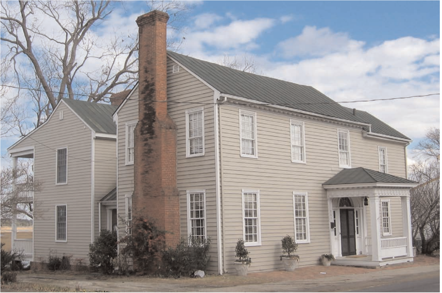
The addition to this residence on South Church Street uses similar materials with simplified details to differentiate it from the original house.
