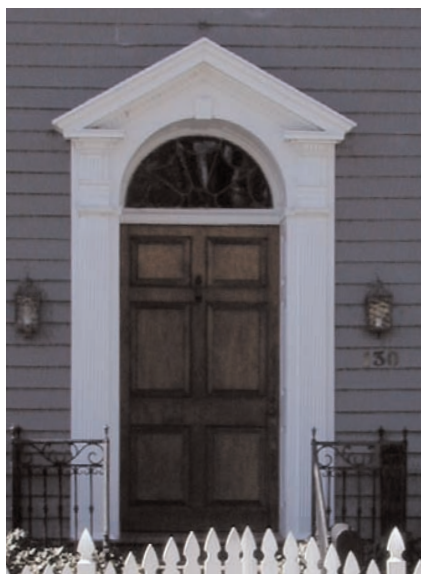
Federal-style entry with six-panel door, applied pilasters and fanlight.
