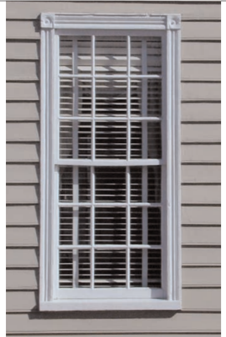
A third treatment found in Smithfield on nine-over-nine double-hung sash is the use of reeded wood trim with decorative corner blocks.
