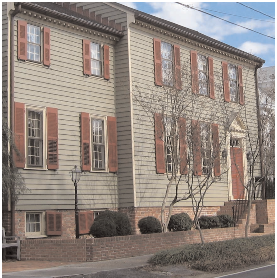
These historic shutters still retain their hardware and are operable, that is they are able to be opened and closed and are not just decoration.
