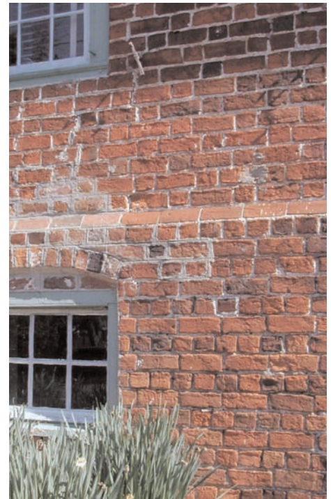
The raised basement is delineated from the first level by a projecting water table.
