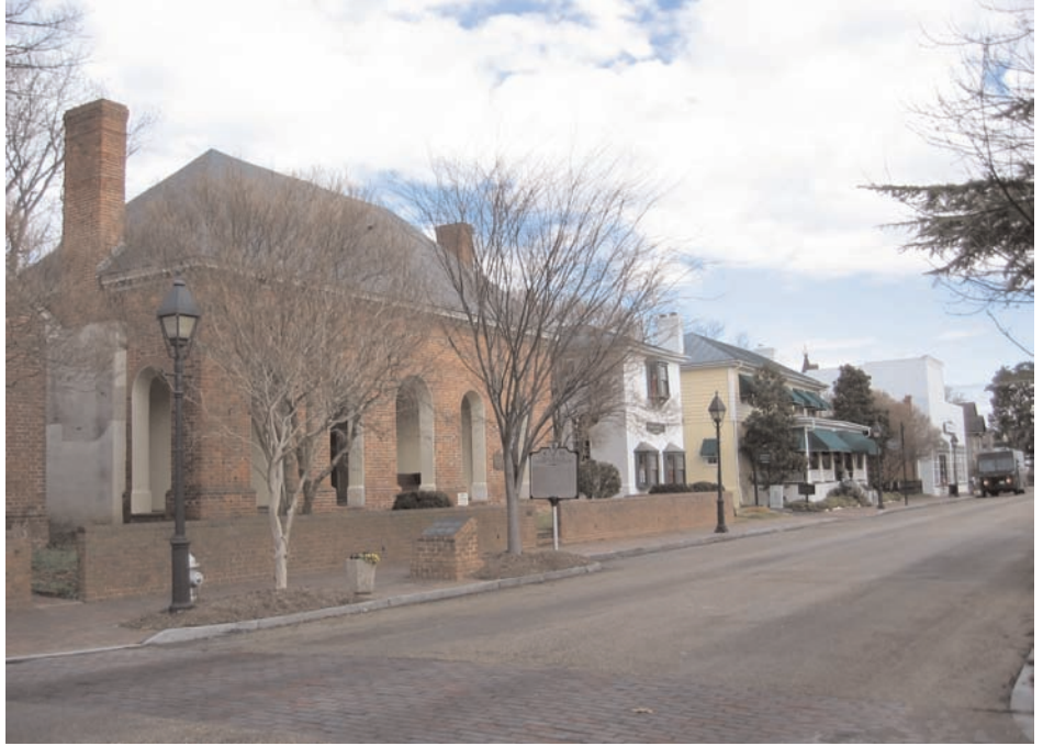
The placement of utilities underground on Main Street highlights the architecture and results in an uncluttered view of the district.
