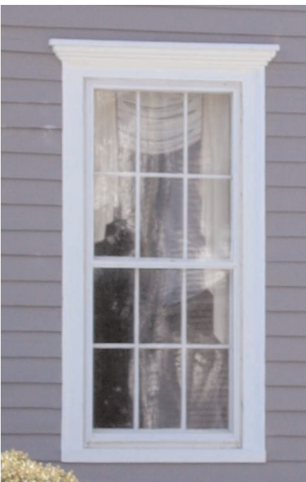
Here, a six-over-six double-hung sash window is capped by a carved wood cornice.
