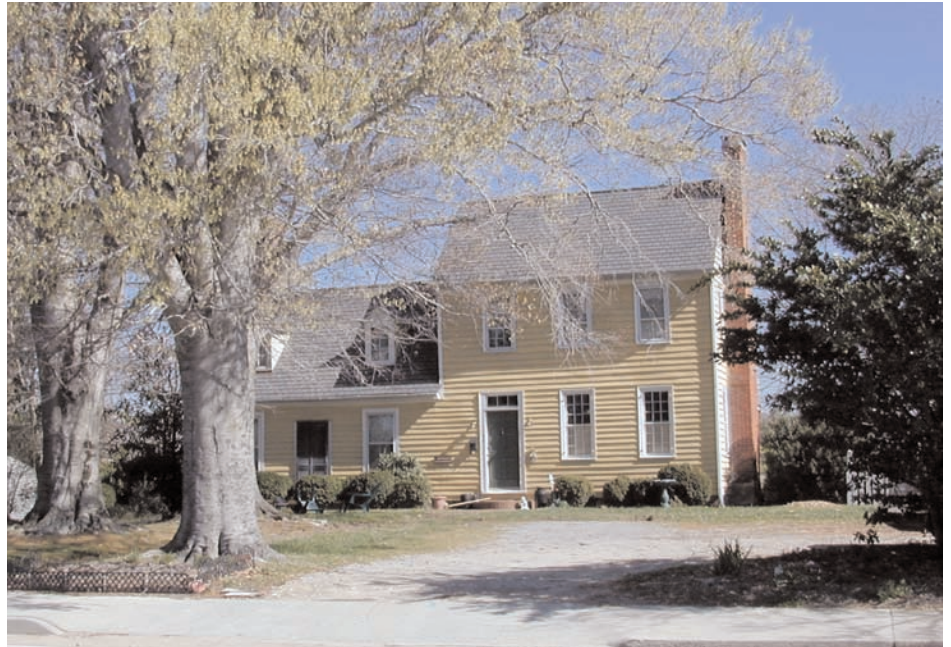
The earlier Georgian, one-and-a-half story portion of this house was updated in the late-nineteenth century with two-over-two windows that give this structure a later appearance. The larger Federal addition retains its original windows.
