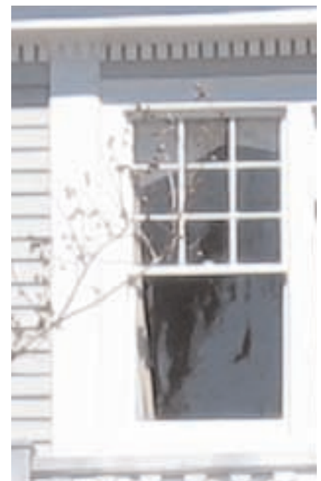
In this Colonial Revival example, a nine-over-one double-hung sash window is surrounded by simple architrave molding.
