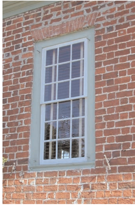
On this example, a nine-over-nine wooden double-hung sash is capped by a brick jack arch.
