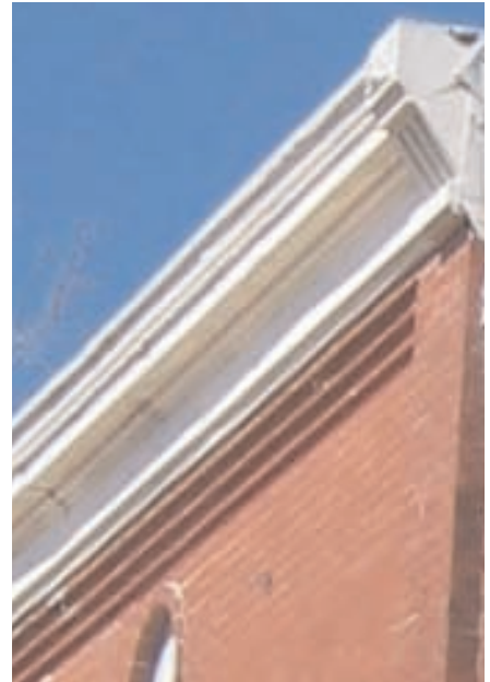
Decorative metal cornice.
