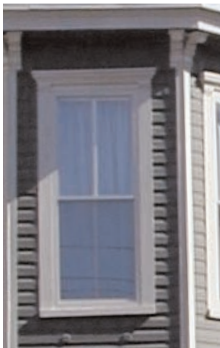
A similar treatment is used on this two-over-two double-hung sash window.
