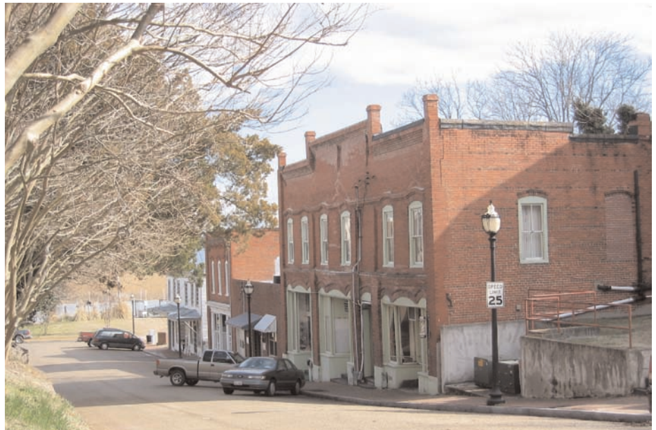
Lower Main Street is commercial/retail oriented and its architectural styles reflect these uses.
