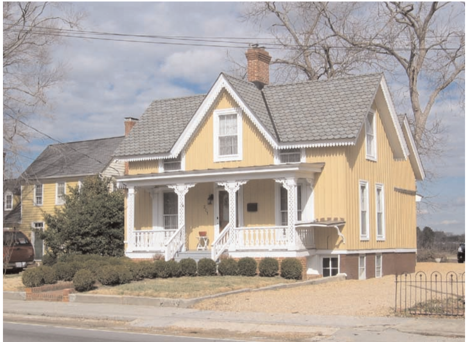
The steeply pitched gable roof covered in fish-scale shingles and gingerbread trim are hallmarks of the Gothic Revival style.
