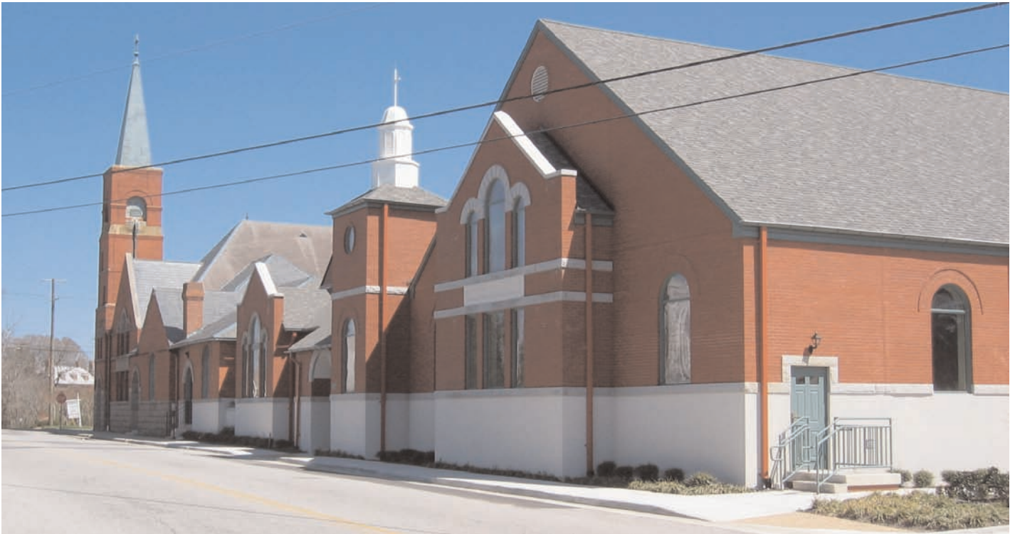
The addition to this church uses massing, scale, materials and architectural features that relate to the original structure but do not replicate it.
