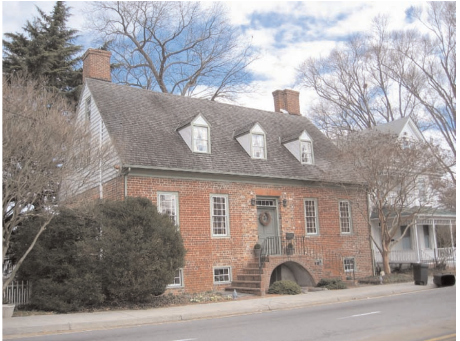
This Georgian one-and-a-half story Flemish bond brick dwelling sits on an English bond raised foundation. The gable ends are clad in weatherboard above the eave line.
