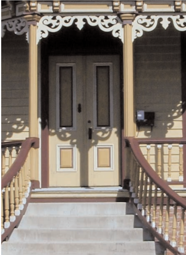
Narrow, paired four-panel doors are frequently found on Victorian houses.
