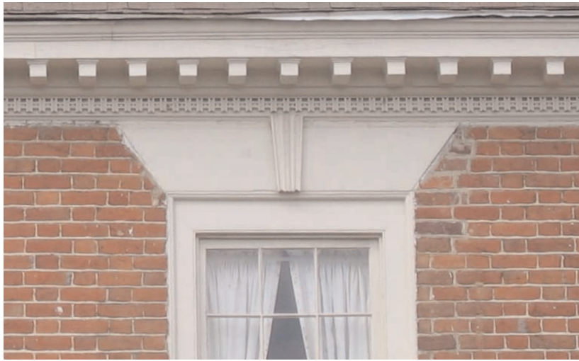
A residential classically decorated cornice with modillion blocks and intricately carved fretwork.
