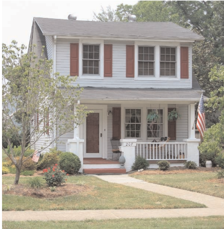
A continuous shed dormer spans the width of this bungalow and echoes the grouped six-over-six windows on the first floor. Short wood columns rest on brick piers to support the full width front porch.
