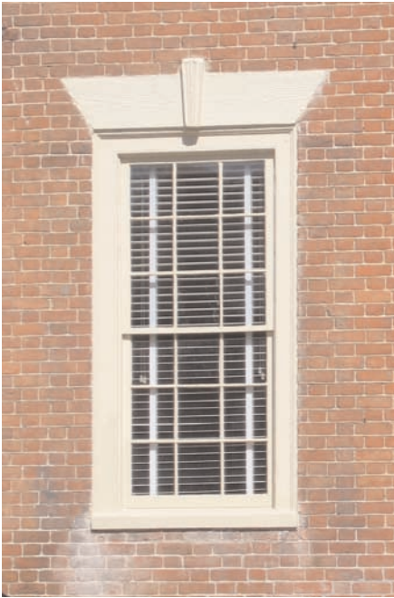
This nine-over-nine double-hung sash is capped by a flat wooden lintel with a carved keystone.
