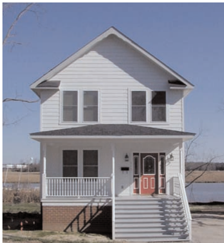
The steep pitch of the gable roof on this new house on South Church Street is appropriate for new construction in the historic district.
