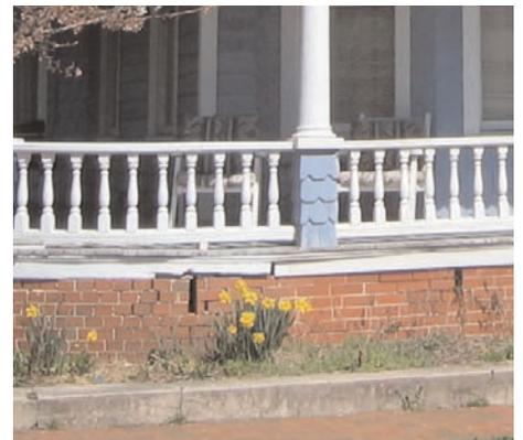
**i** Most foundations in Smithfield are of masonry. Brick piers are the most common and distinctive foundation type, especially for vernacular frame houses; many have been filled in with solid brick or concrete block; a few houses have stone foundations.
